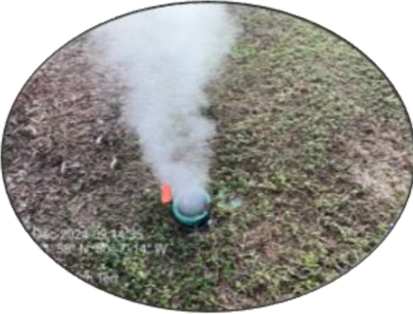
Cleanout Riser Replacement
