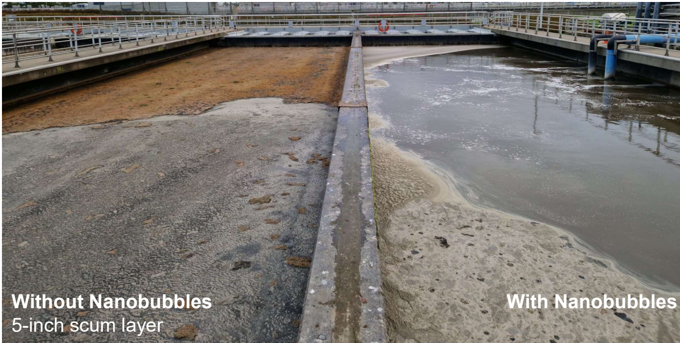
Primary Clarifiers Copenhagen, DK
